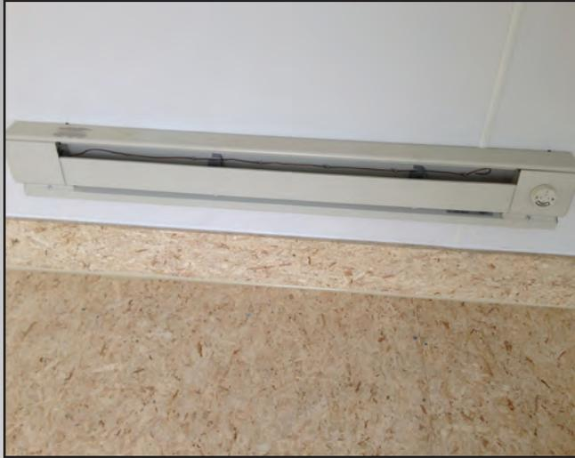
**BASEBOARD HEATING SYSTEM** - A must for the year-round roving workshop. The self-contained unit comes with an optional adjustable thermostat control or wall-mount thermostat.
